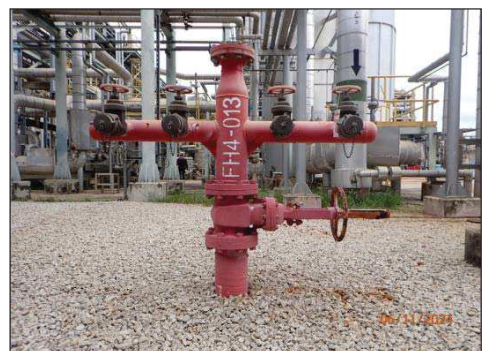
Fire Hydrant/Monitor
